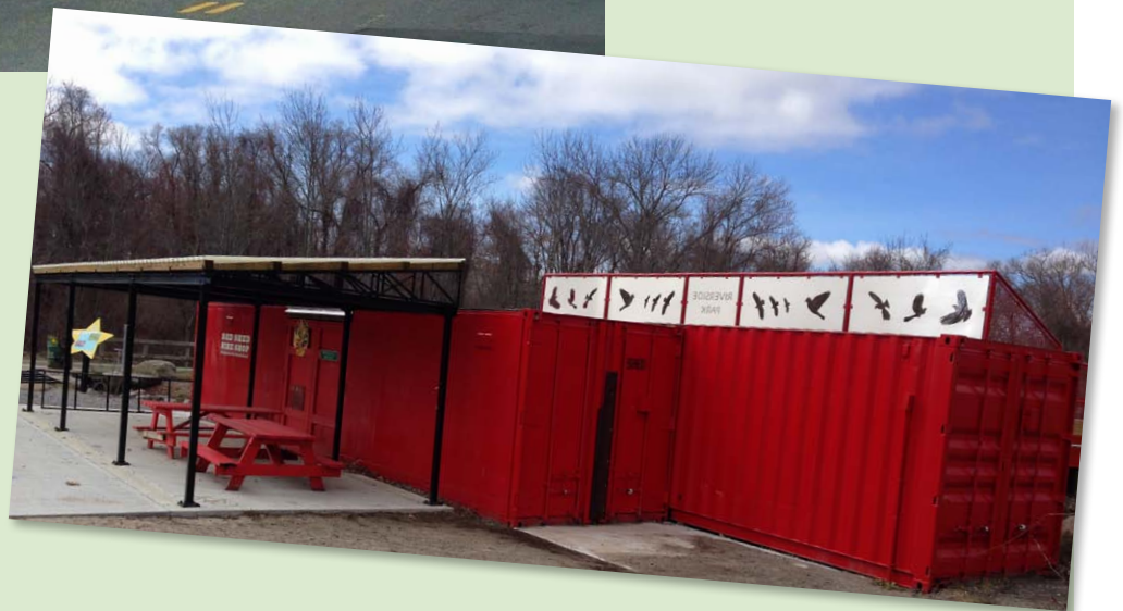
Right: The Red Shed Bike Shop at 50 Aleppo Street in Providence will have a green roof installed this summer with 160 vegetated shortgrass modules that will retain and filter over 700 gallons of stormwater.
