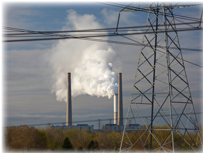
DTE Energy’s coal-fired power plant in Monroe Michigan is among the worst polluters in the country.
