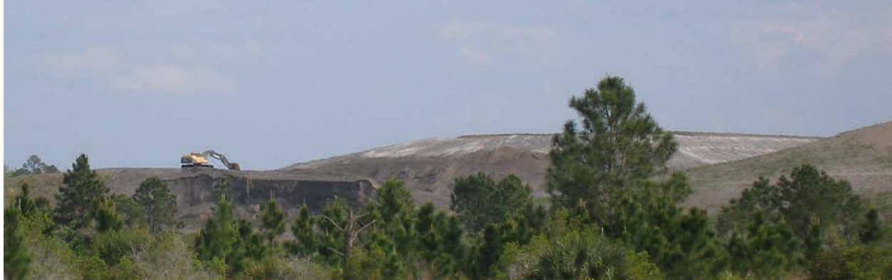
Photo Coal ash landfill at Stanton Energy Center Photo Credit: Angelique Giraud February 2012
