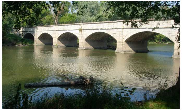
The Monocacy Aqueduct.
