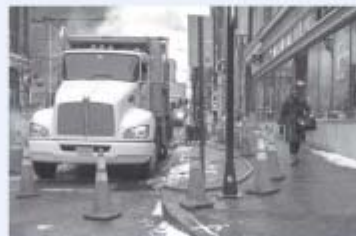
Water main repair at W. Baltimore Street & N. Howard Street.
