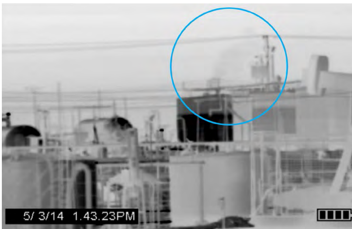
Emissions rising from a processing facility in the Lost Hills oil field. Note the blue circle indicating a plume. These emissions cannot be seen without the assistance of the FLIR infrared camera.
