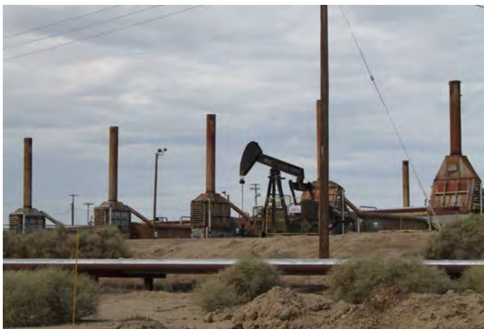
At the same processing facility taken on the same day within minutes of the picture above, emissions are invisible without the FLIR camera.
