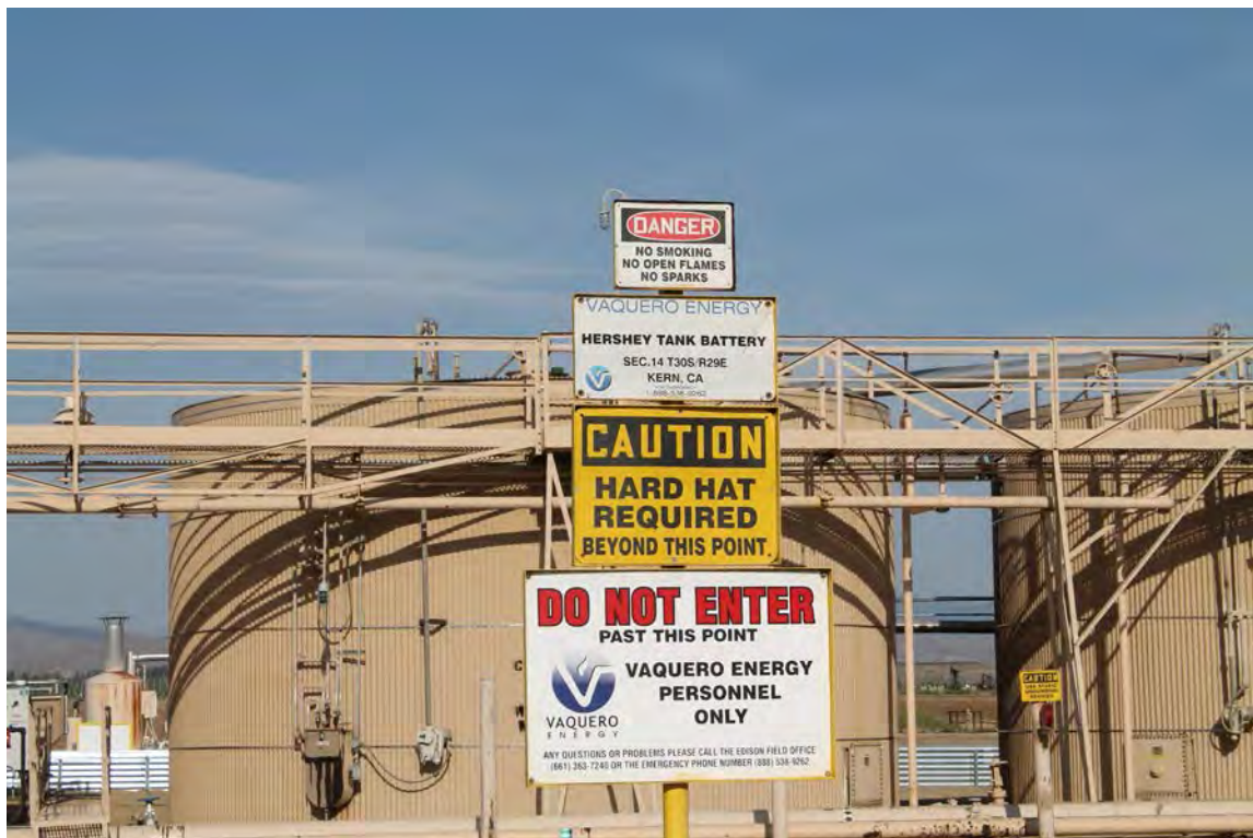
Storage tanks are typical sources of VOC (Volatile Organic Compound) emissions.
