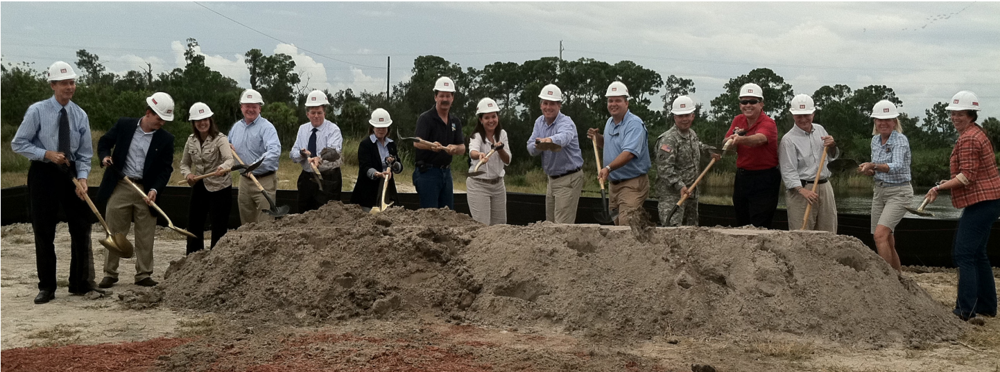
Local officials and conservationists, including U.S. Rep. Tom Rooney (far left) and South Florida Water Management District Executive Director Melissa Meeker (far right), gather for the October 28, 2011 groundbreaking ceremony on the C-44 Reservoir and Stormwater Treatment Area in Indiantown, Florida.
