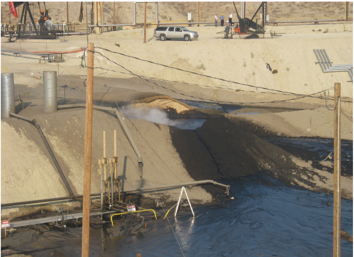
Chevron Well 20, where a thermal enhanced oil recovery blowout at the Midway-Sunset Oil Field, Kern County, California occurred. In June 2011, a Chevron construction supervisor died when a known surface expression from a steam injection operation expanded into a sinkhole, expelling steam, oil and wastewater to the surface.
